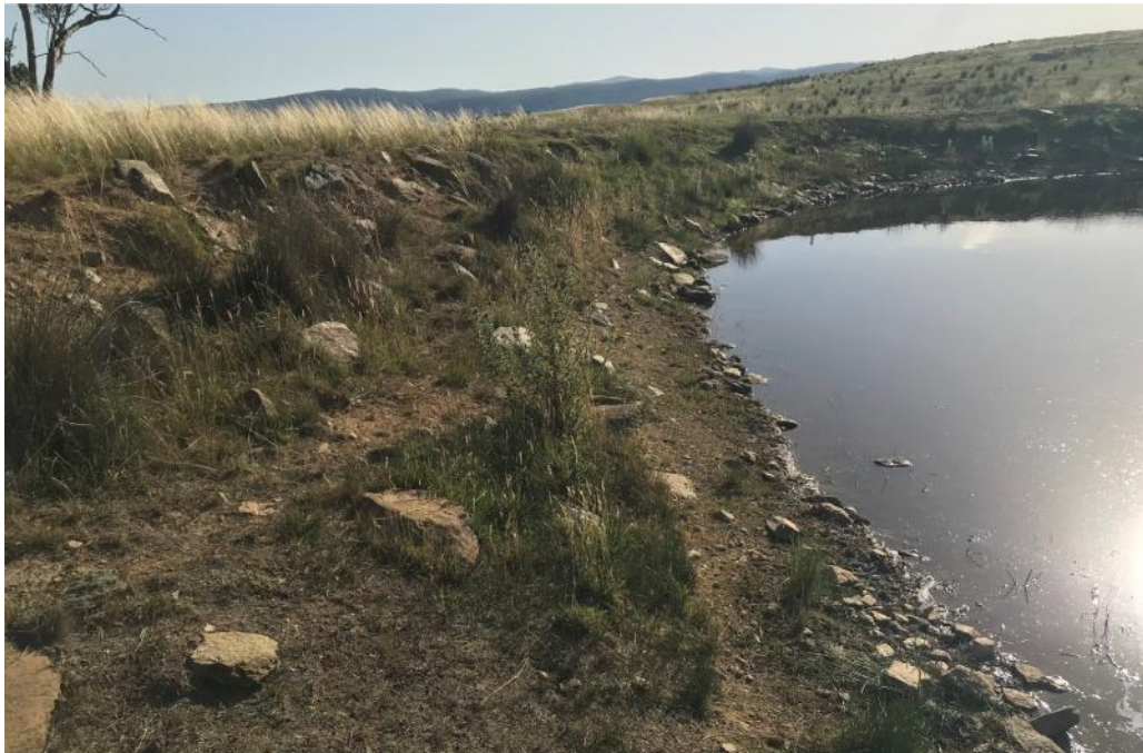
Photo A30 – Boulders in dam embankment filling. Refer Drawing 2 for locality and direction
