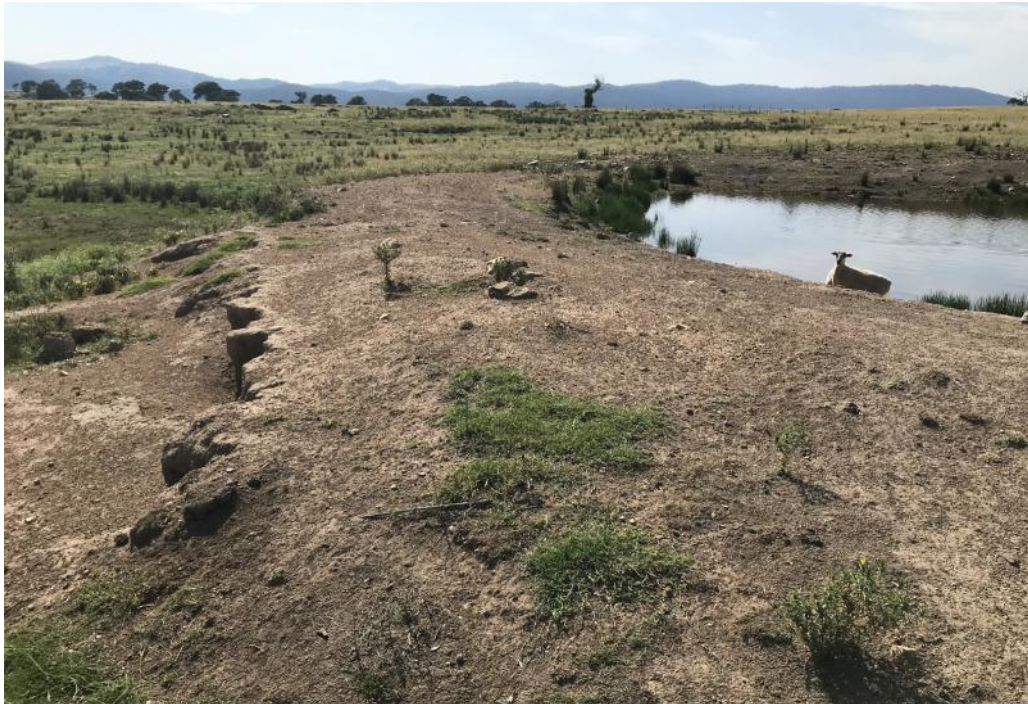
Photo A39 – Erosion in dam wall. Refer Drawing 2 for locality and direction
