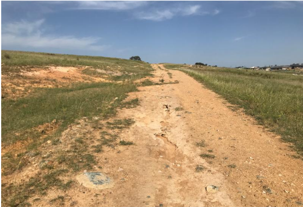
Photo A37 – Erosion in access track and hill side. Refer Drawing 2 for locality and direction
