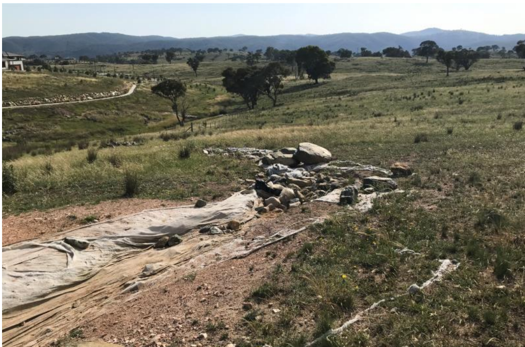
Photo A36 – Geofabric lined swale drain with boulders. Refer Drawing 2 for locality and direction
