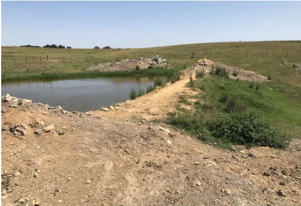
Photo A49 – Recently placed weathered rock at dam abutments. Refer Drawing 2 for locality and direction
